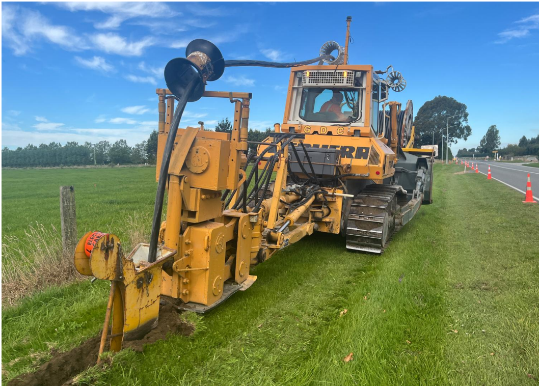
Mole ploughing Methven Highway (completed April 2026)
